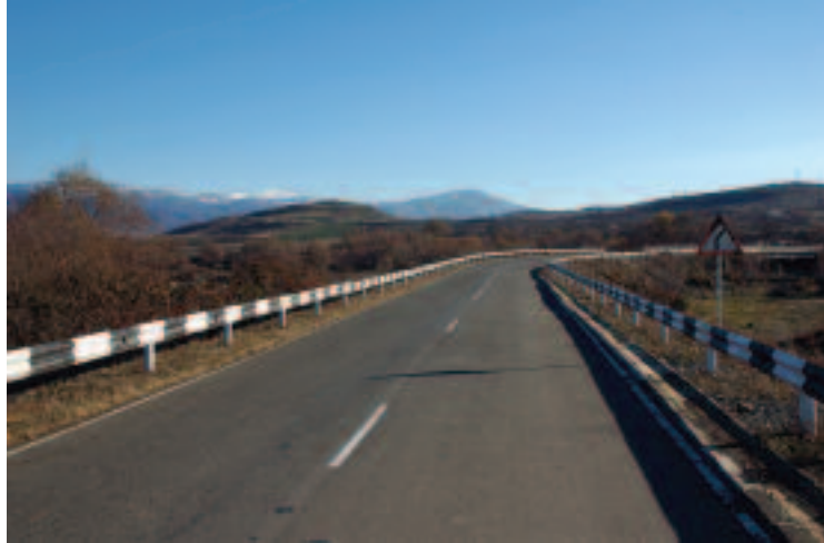
North-South Highway — the "Backbone of Karabakh"
